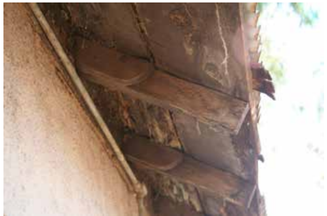
South Eave Close up
