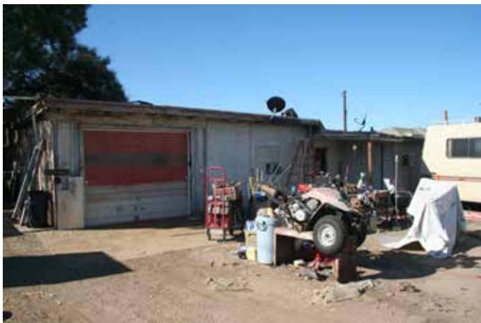
House Addition to North West
