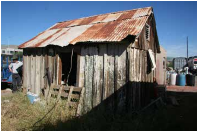
Shack Overview to North West
