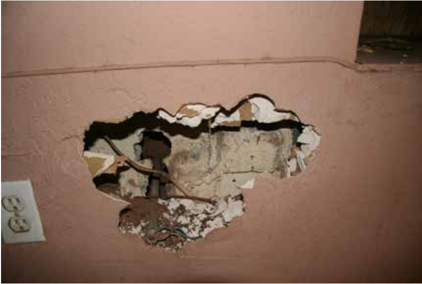
Adobe Wall base at South
