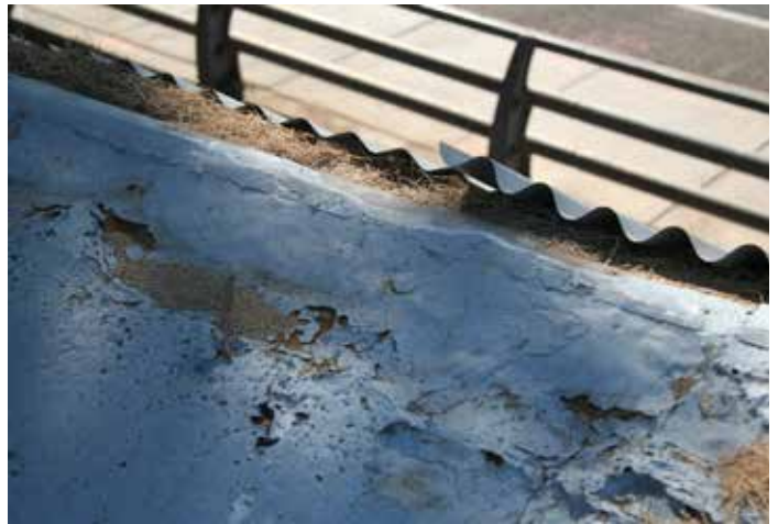
Roof Ridge Closeup
