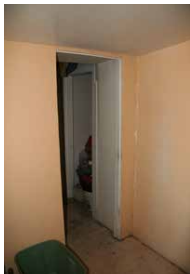
Door 7 Interior View
