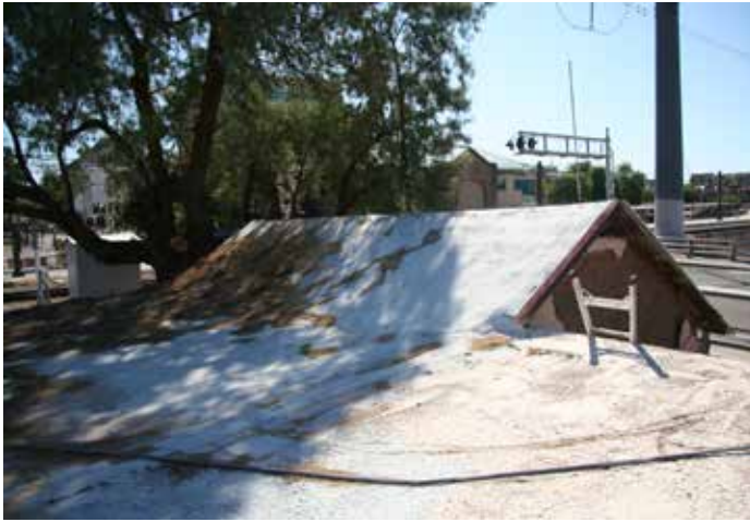
Roof to South East
