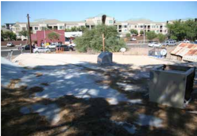
Roof to West
