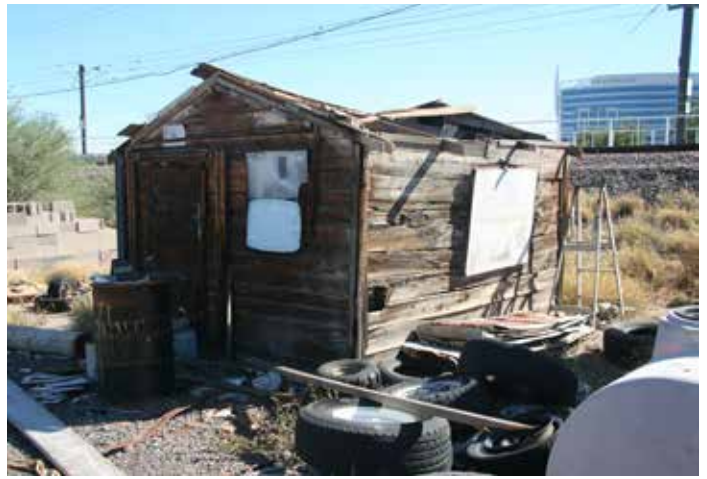
Cabin Overview to South West
