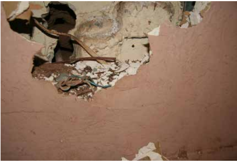
Adobe Wall base at South
