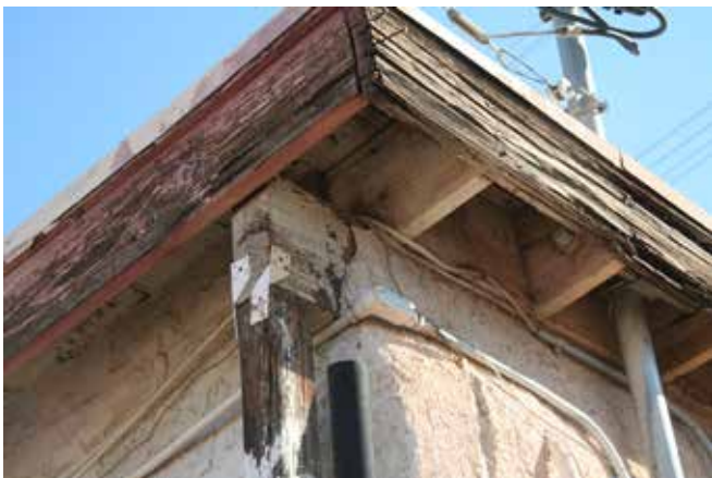
Eave at South West Corner
