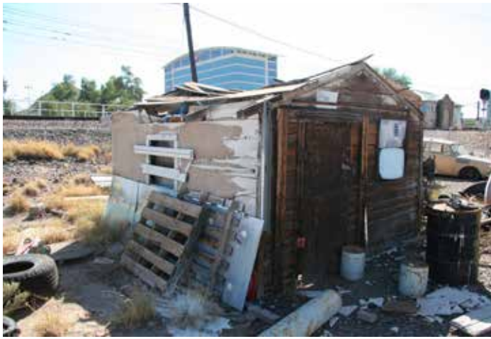
Cabin Overview to South East
