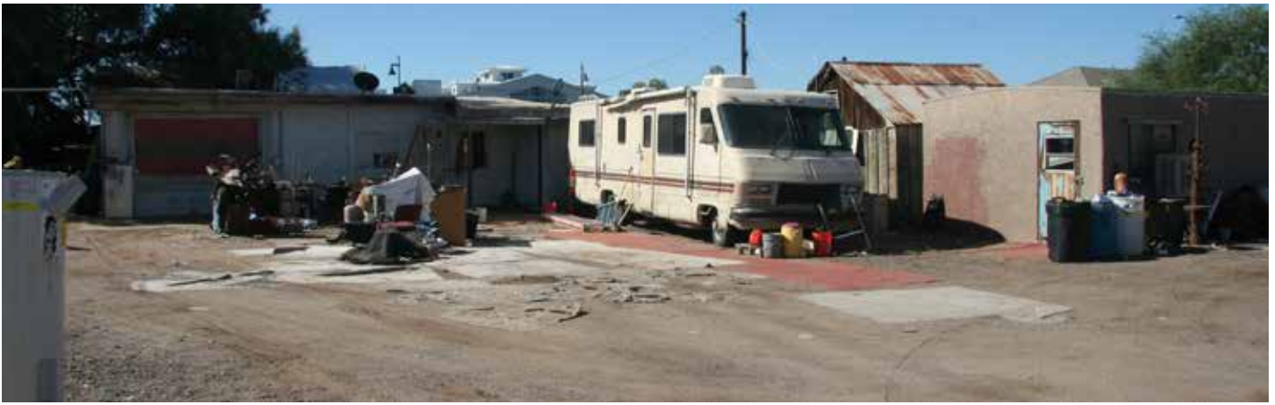
Overall view to southwest. Shack (with metal roof) at right
