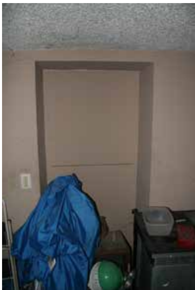
Door 6 Interior View
