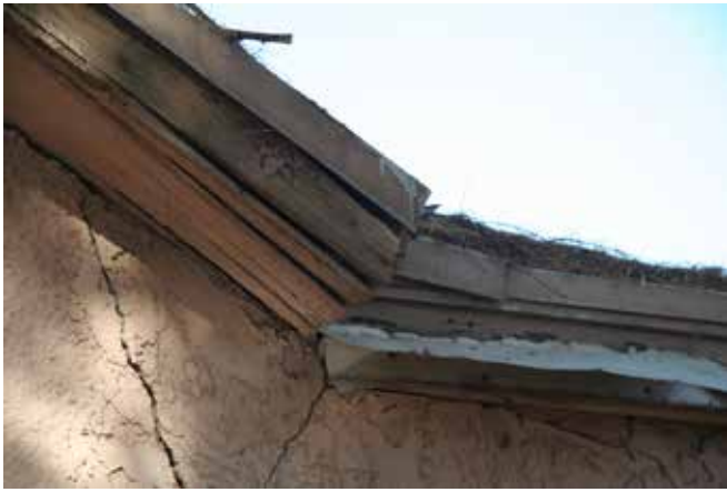
East Fascia at Joint
