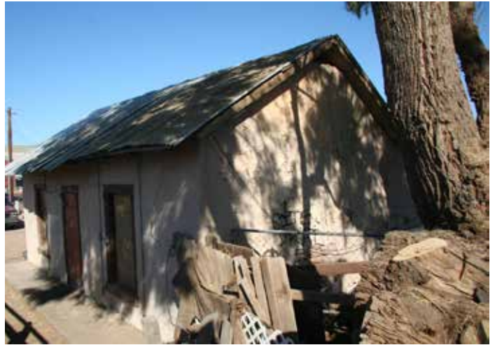
View to North West
