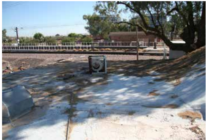
Roof to East
