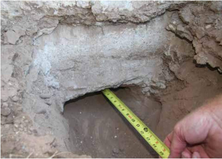
Adobe foundation excavation
