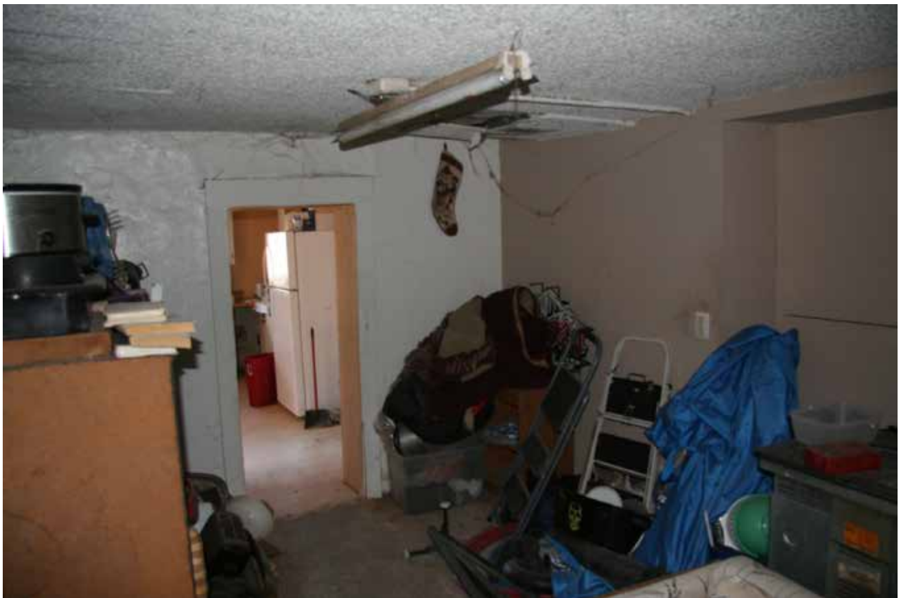
Interior, Room 3, looking northeast
