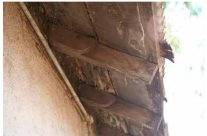
South Eave Close up
