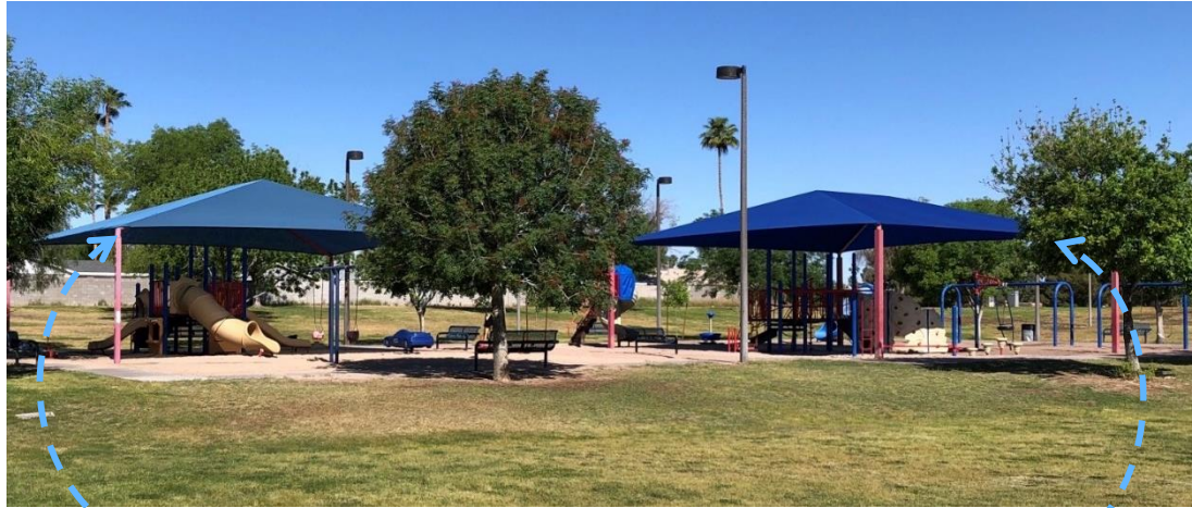
Playground Shade Structures to be Replaced
