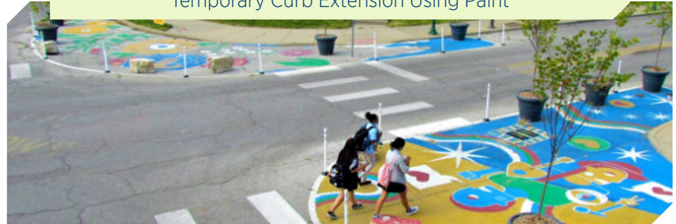
Temporary Bulb Out and Painted Crosswalk
