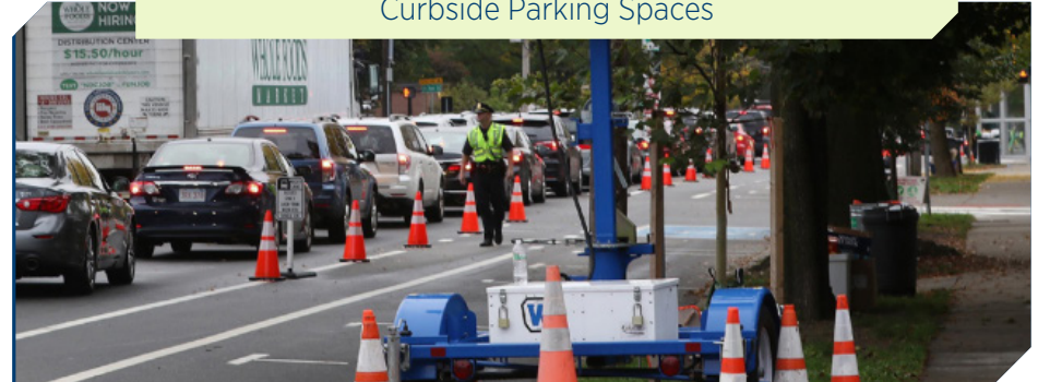
Temporary Transit Lanes Accomplished by Adapting Curbside Parking Spaces
