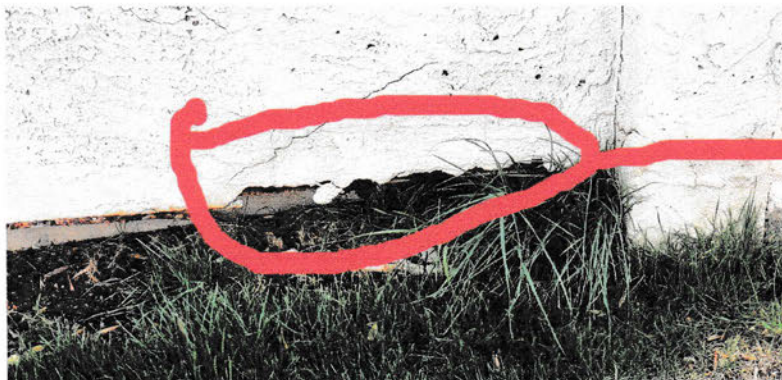
Wall damage resulting from watering grass adjacent to wall
