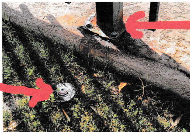
New pool fence rusting from adjacent grass over spray
