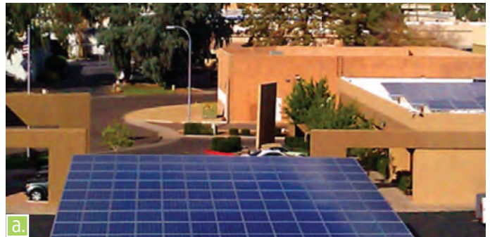
A great community example is Tempe Solar Park at The 6th Street Commercial Center which has panels installed on the building’s roof, a parking shade structure made primarily of panels, and panel-covered exterior walkways (top).
