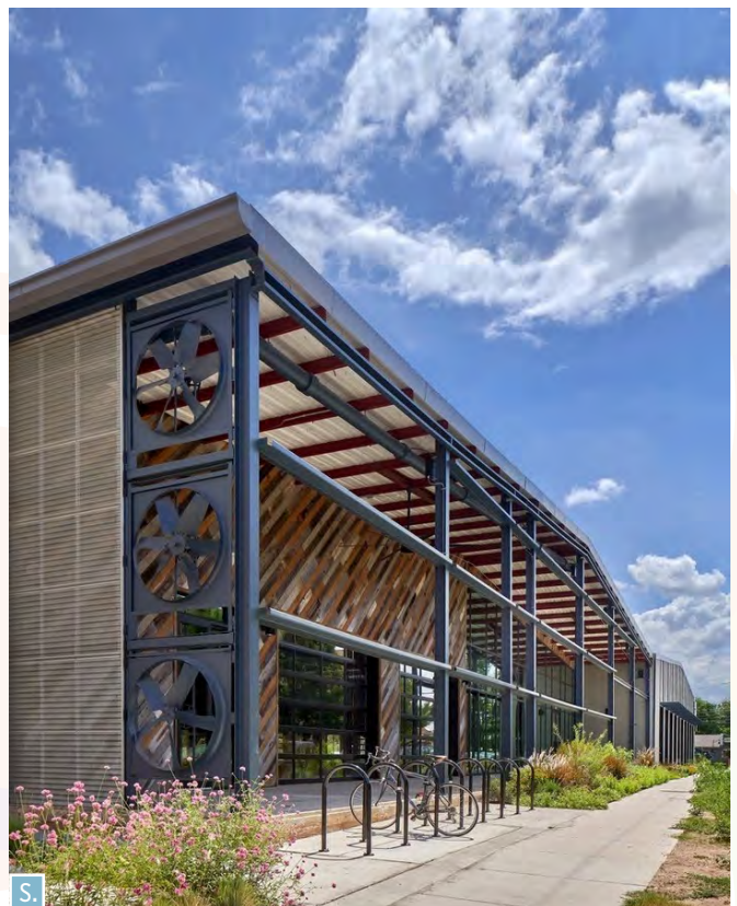
This project managed to reuse 95% of the existing building, including the building skin, which was turned inside-out to reveal the original metal finish and industrial exhaust fans that were used as decorative details (above).
