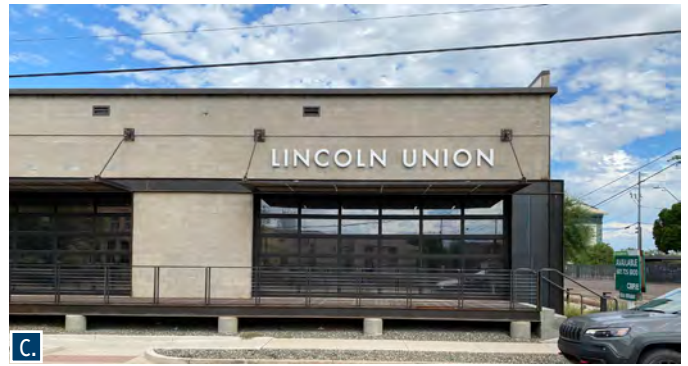
Architectural features along highly visible street frontages can enhance the overall gateway experience (above).
