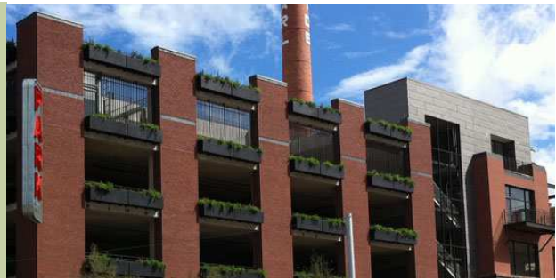
Planter boxes at install
