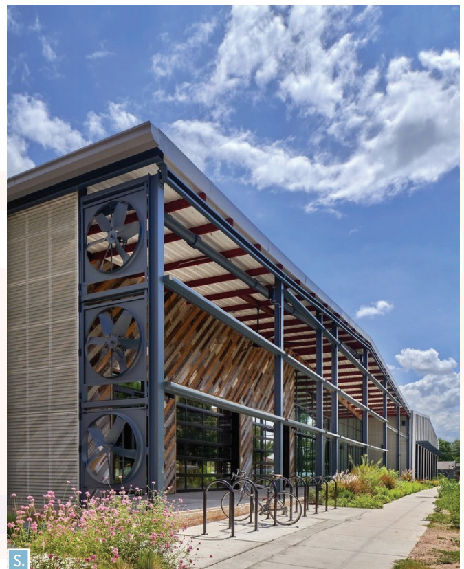
This project managed to reuse 95% of the existing building, including the building skin, which was turned inside-out to reveal the original metal finish and industrial exhaust fans that were used as decorative details (above).
