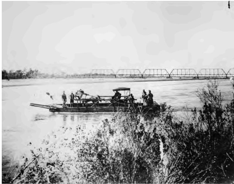
fig. (7) Crossing the Salt River HABS HAER 29-2 before the bridge. ca. 1912
