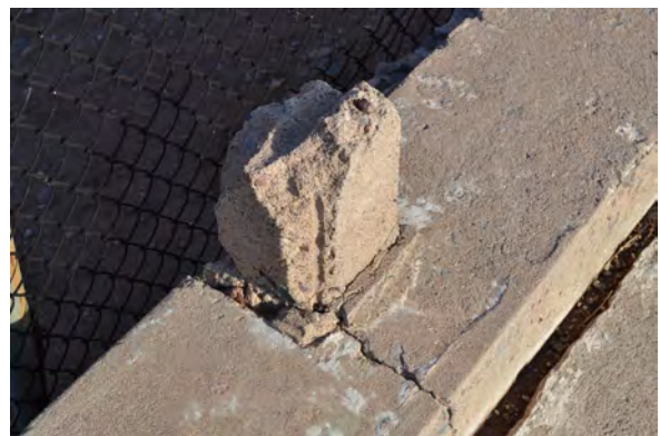
fig. (28) Remaining piece of historic bollard on west curbing. Note gap between road and curb. Photo 2018.
