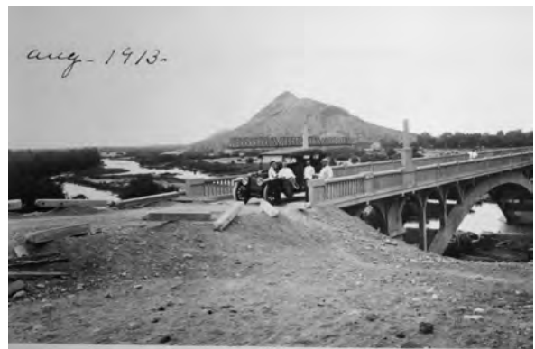
fig. (27) HABS HAER photo ca. 1913 showing Ash Ave Bridge west side bollard installation.
