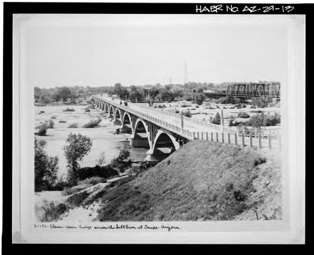
fig. (5) Tempe Ash Avenue Bridge from north bank, ca. 1913, HABS HAER archives collection. HAER no. AZ-29-13.
