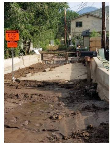
Monsoon storms resulted in significant runoff of debris and stormwater, which blocked stormwater conveyance systems and resulted in severe flooding.
