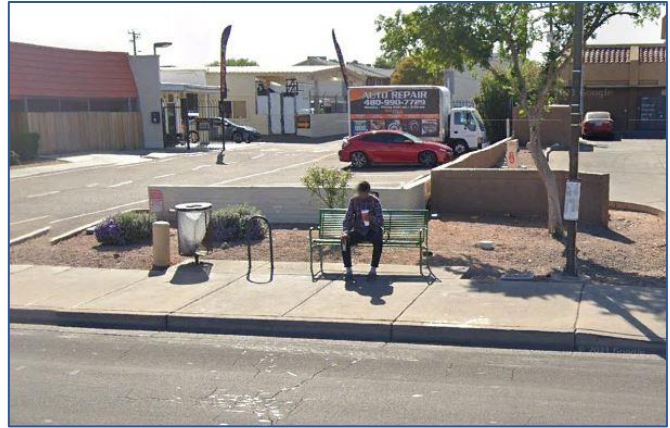
Unsheltered Bus Stop (Southwest Corner of Scottsdale Rd. and Continental Dr.)
