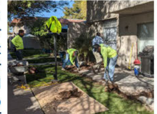
Footings for a patio wall.
