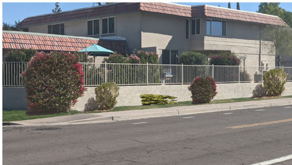
Plantings along Southshore Wall just West of Signage
