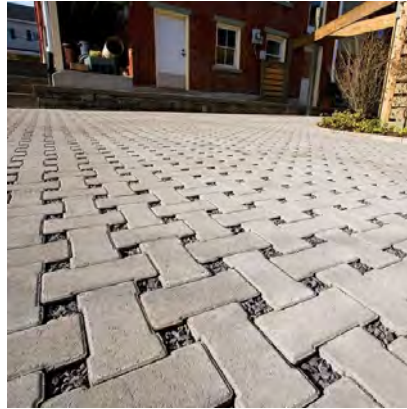
Permeable Pavement Surfacing that allows for surface-water penetration and filtration
