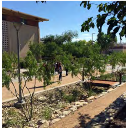
Vegetated Swale Linear landscaped bio-retention areas capture surface storm-water from adjacent paved surfaces
