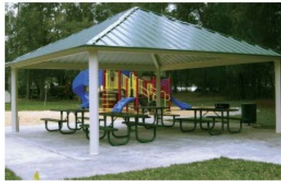
PICNIC AREA RAMADA METAL ROOF STRUCTURE
