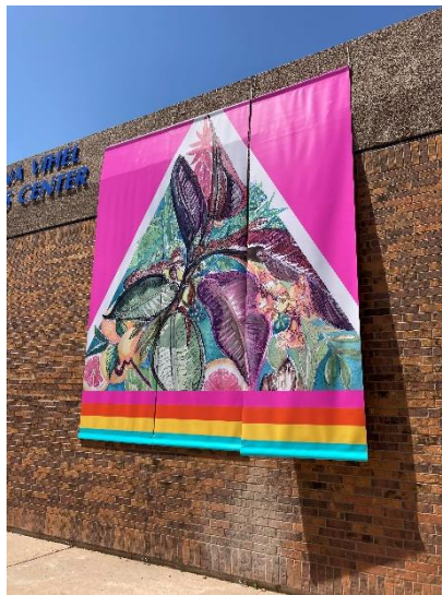
Exterior banner being installed
