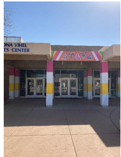
Columns being painted during installation
