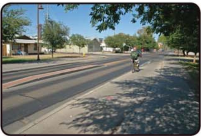
Ramped Bike Lanes
