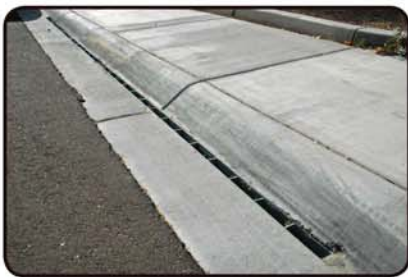
Rolled Curb & Stormwater
