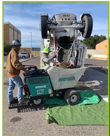
Lawn Area Concrete
