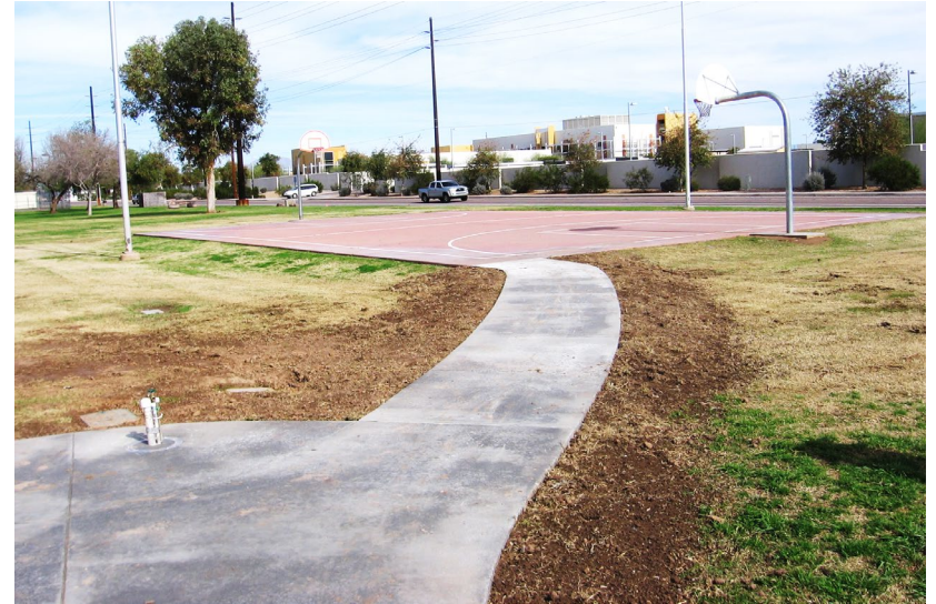
Indian Bend Park - ADA compliant walkway
