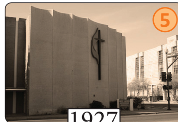
First United Methodist Hall 215 East University Drive
