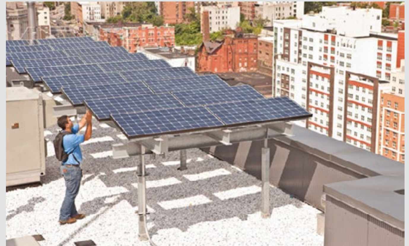
Installation of RPH solar photovoltaics on NYC building (Source: NYCEDC)
