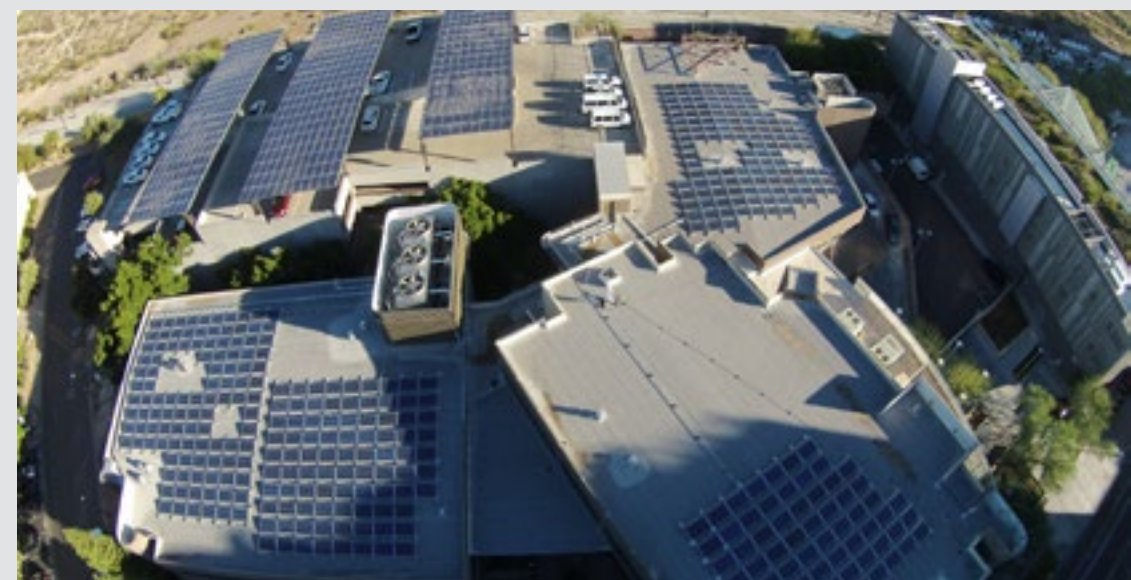
Solar panels on Tempe Police Department building (source: City of Tempe)
