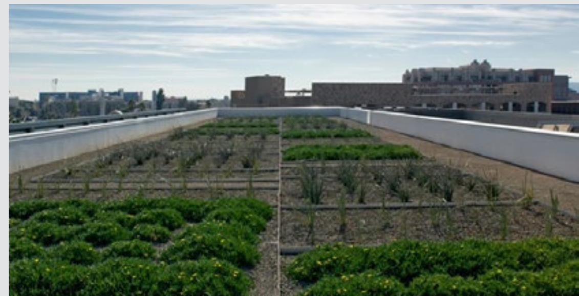
Garden rooftop and cool materials (source: City of Tempe)
