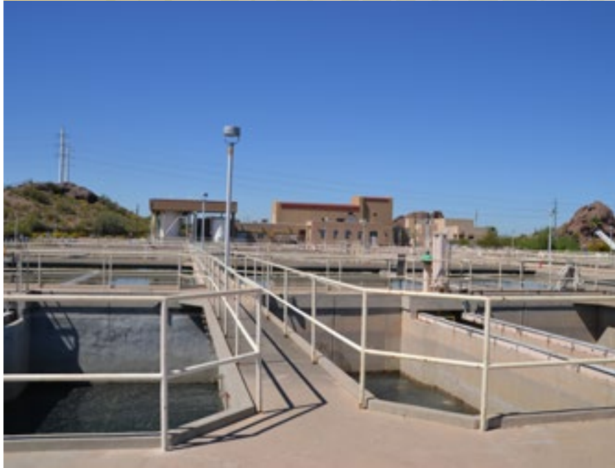
JGM Water Treatment Plant (source: City of Tempe)
