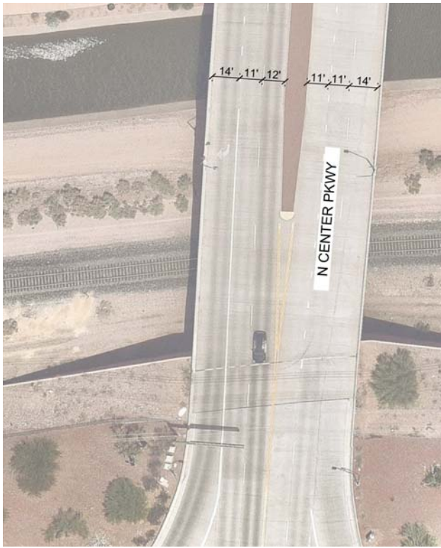
2 N. CENTER PKWY - EXISTING CONDITIONS
