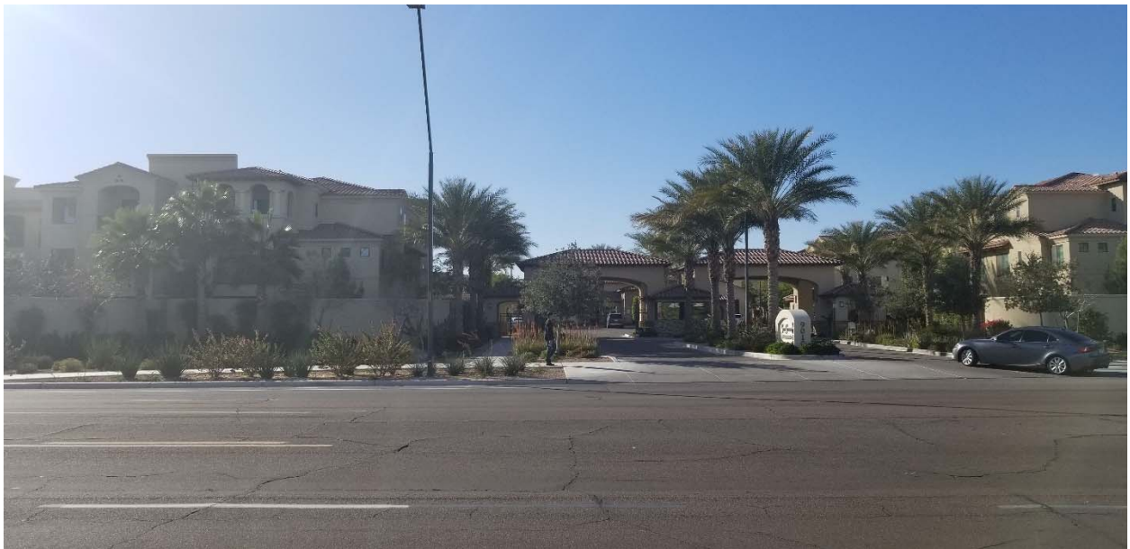
NWC looking West
