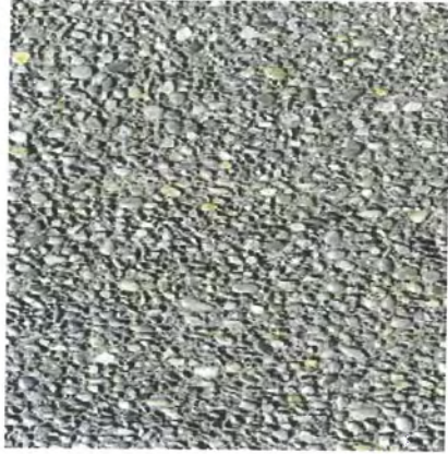
EXPOSED AGGREGATE CONCRETE WALL
