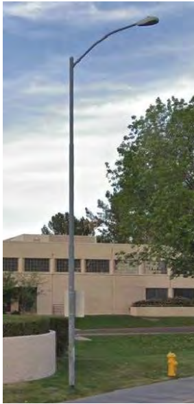
EXISTING COBRA LIGHT ALONG CURRY TO BE RELOCATED
