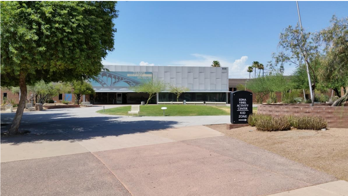
Site Photo 6 - Tempe Public Library
