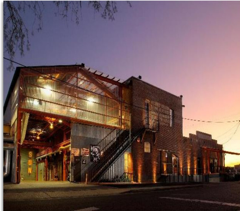
New look of ASU Grant Street Studio – Phoenix, AZ Adaptive reuse of manufacturing space to artist studios and gallery
