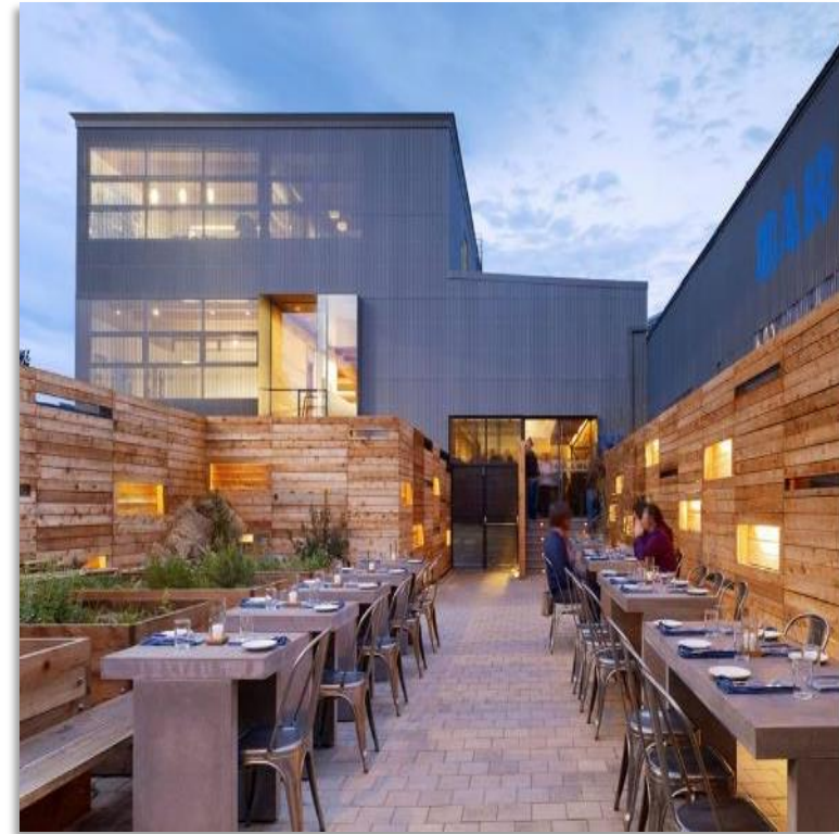
Adaptive reuse of historic industrial building to a restaurant and office. LEED Gold. 355 11 th St., San Francisco, 2008
