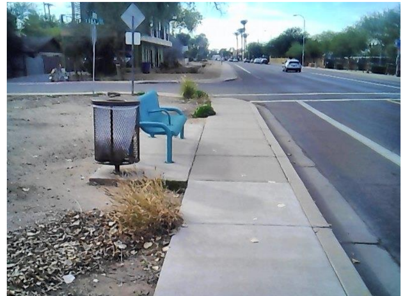
Expand Bus Pad Landing
