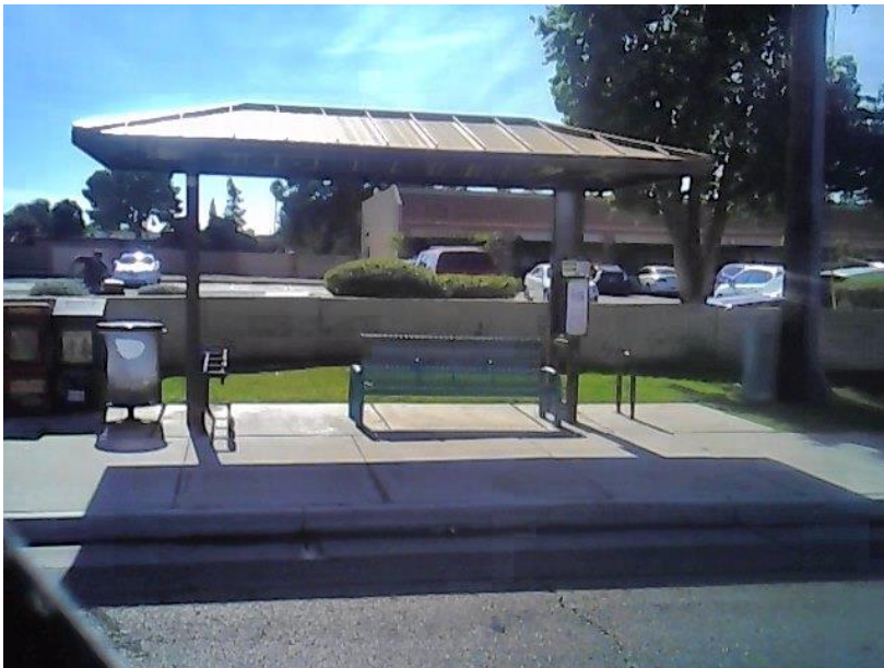
Compliant Transit Stop
