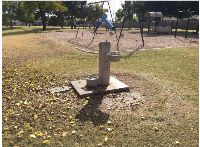
Drinking fountain with no accessible route.
