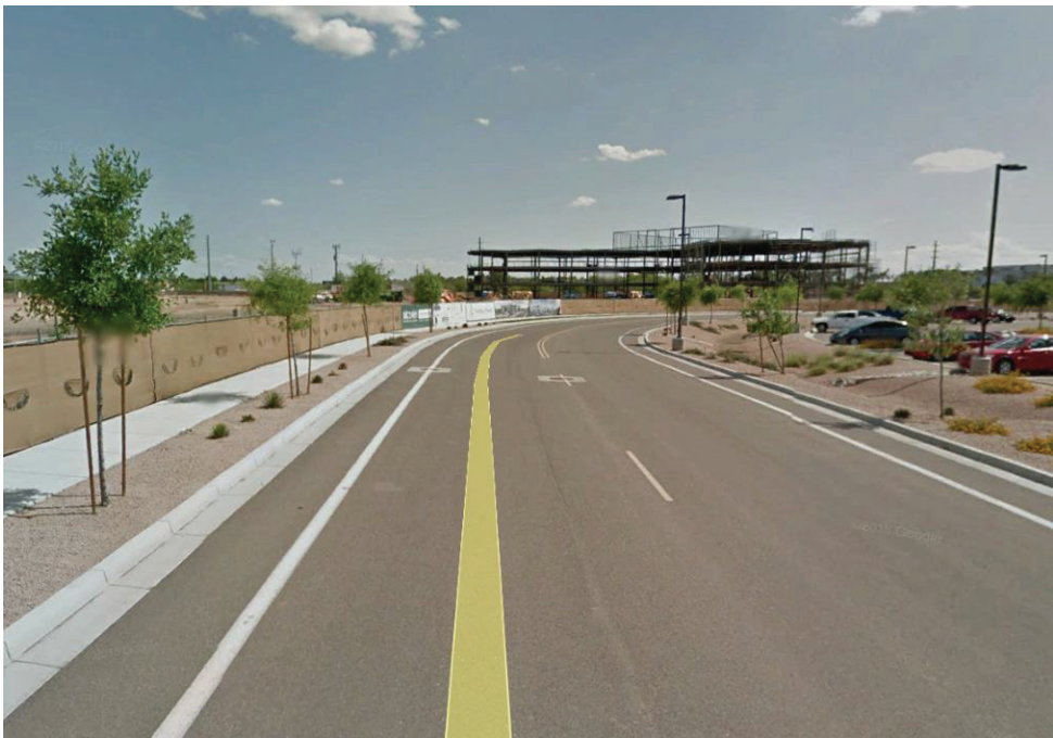
11. Location C (SWC) facing south
