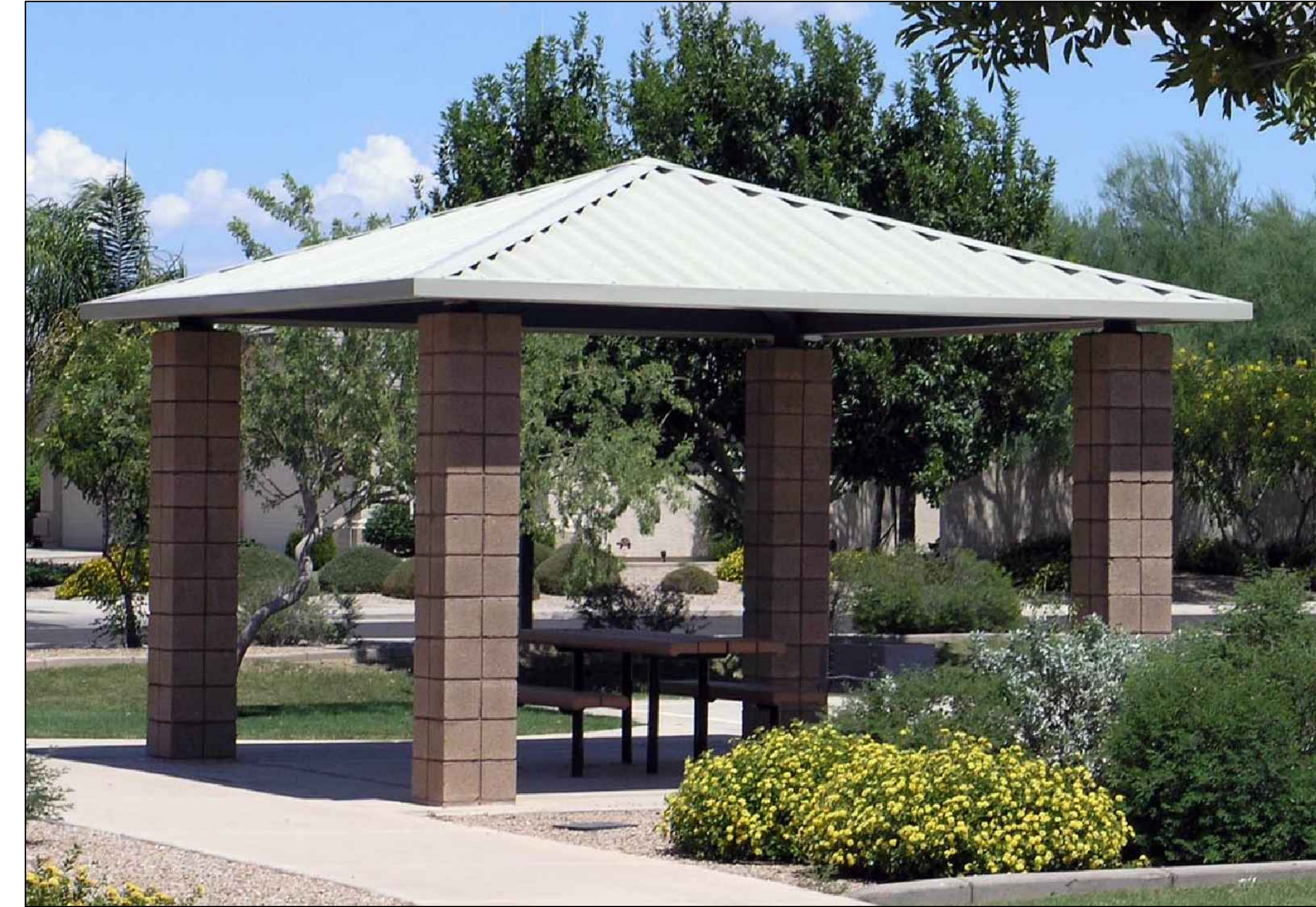
SCoured CMU BLOCK FINISH
