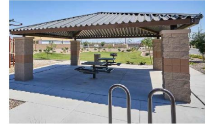
PICNIC RAMADA METAL ROOF STRUCTURE
