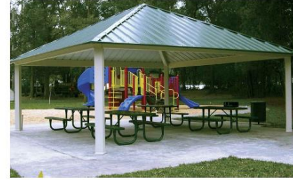
PICNIC RAMADA METAL ROOF STRUCTURE
