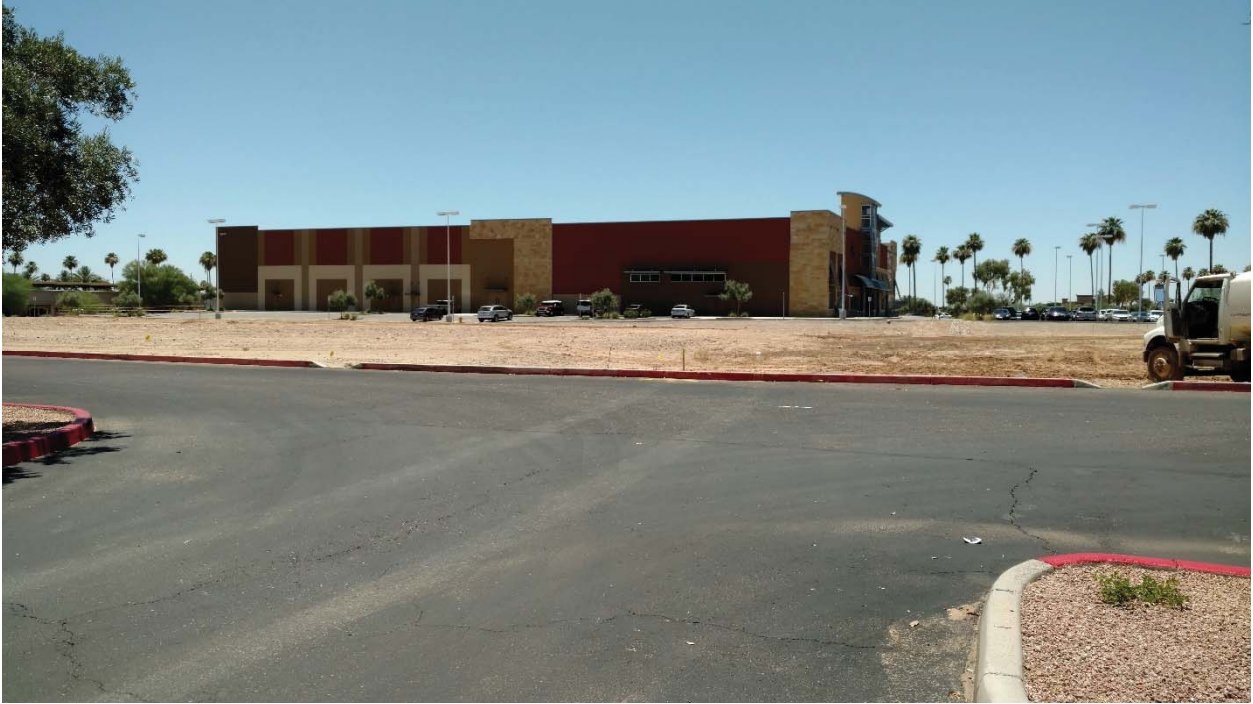
9. Looking south at property.
