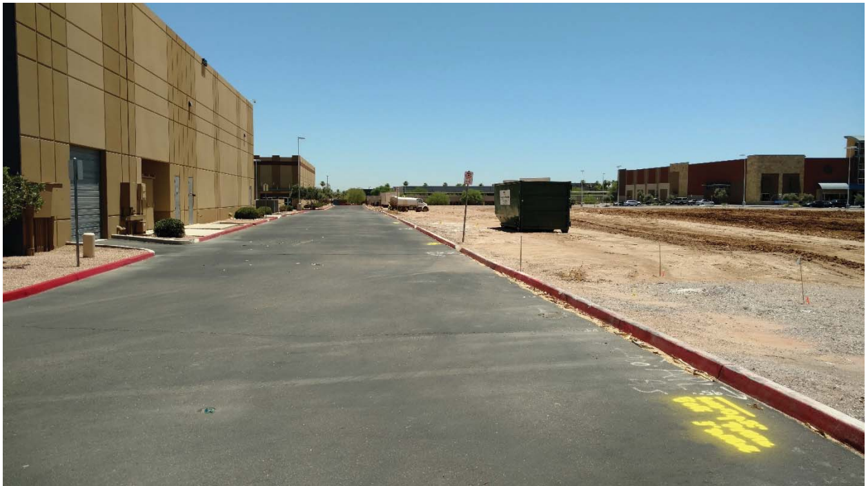
8. Looking east from north side of property.
