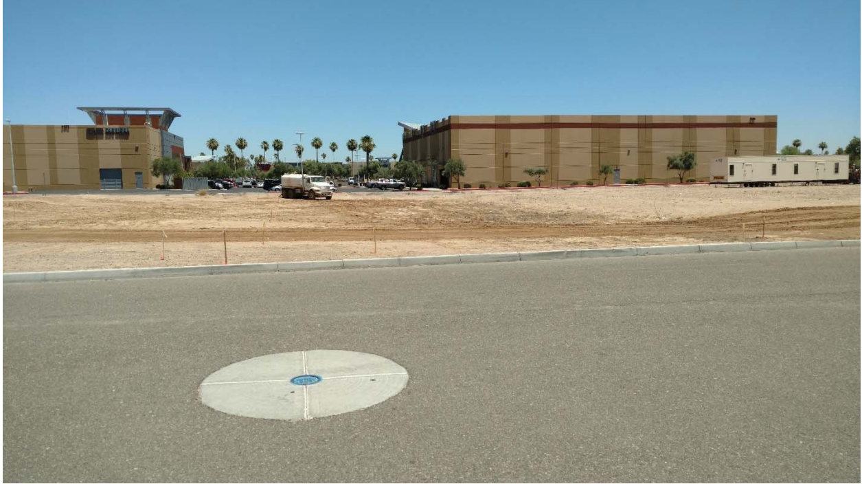
7. Looking north to adjacent buildings.
