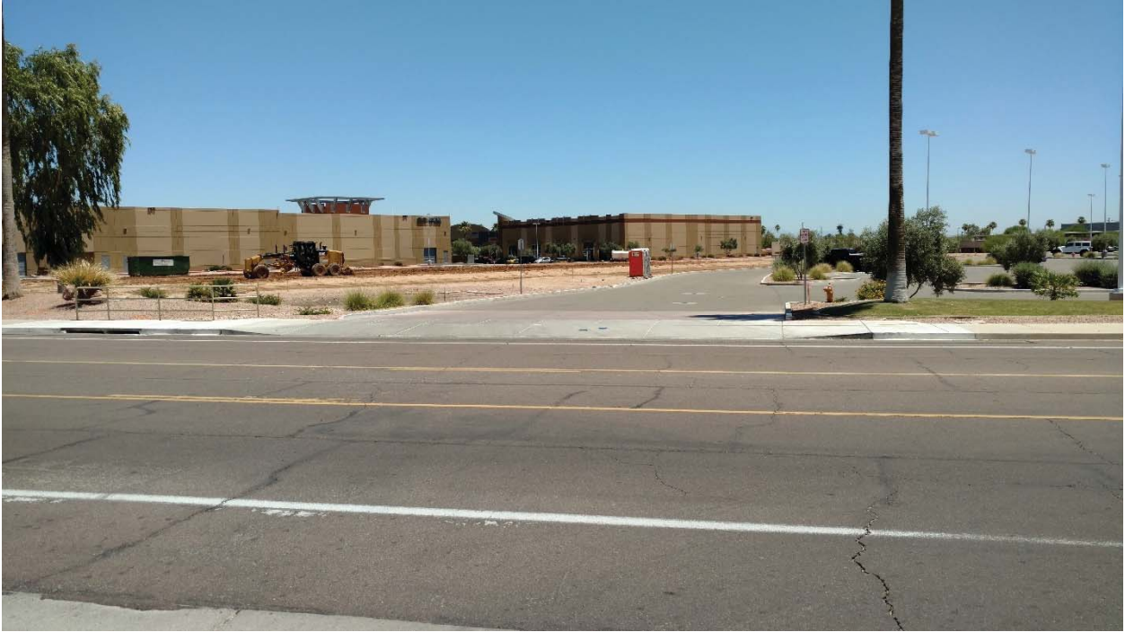
3. Main driveway into site from Emerald Drive.
