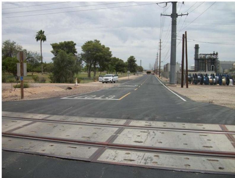
Missing Link connection at approved railroad crossing, SRP drive and golf course access (facing east)
