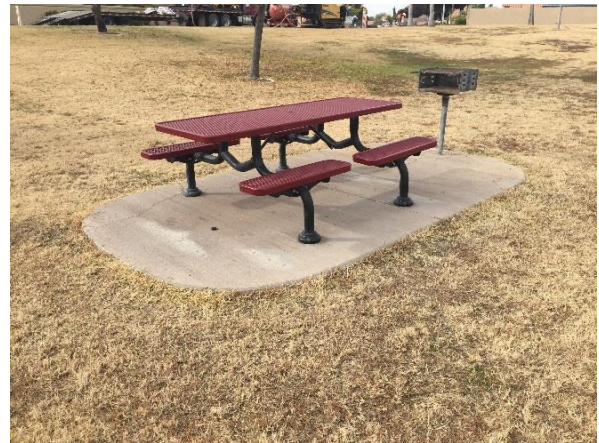
Figure 28: Corbell – Ex: No accessible route to amenities
