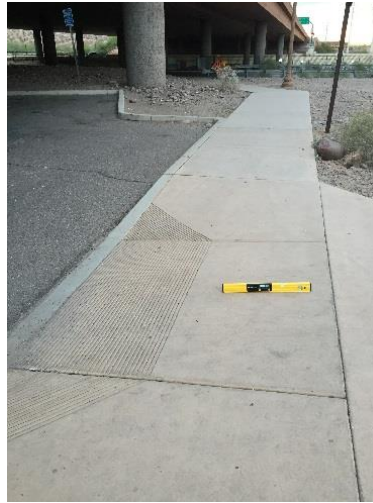
Figures 25 and 26: Curb ramp slope 10.9%
