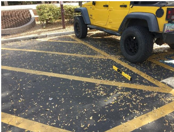
Figures 15 and 16: City Hall West – 4.0% slope within space and aisle
