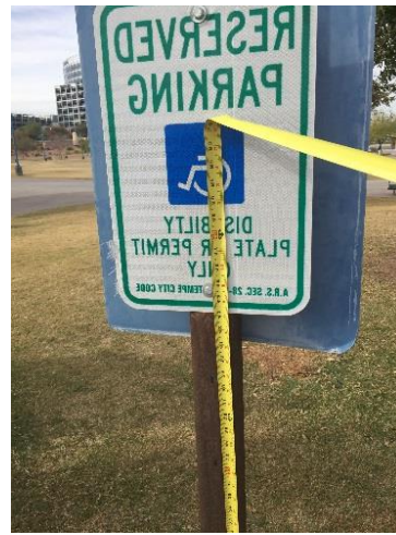
Figure 18: Parking signs are too low.
