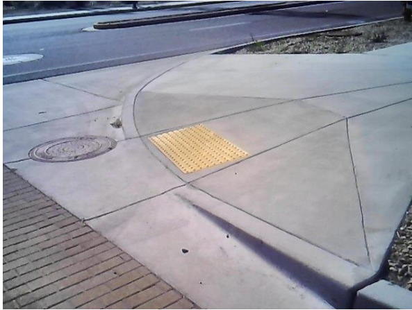
Figure 2: Compliant Perpendicular Ramp Figure 3: Needs truncated domes
