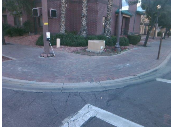
Figure 2: Compliant Perpendicular Ramp Figure 3: Needs truncated domes
