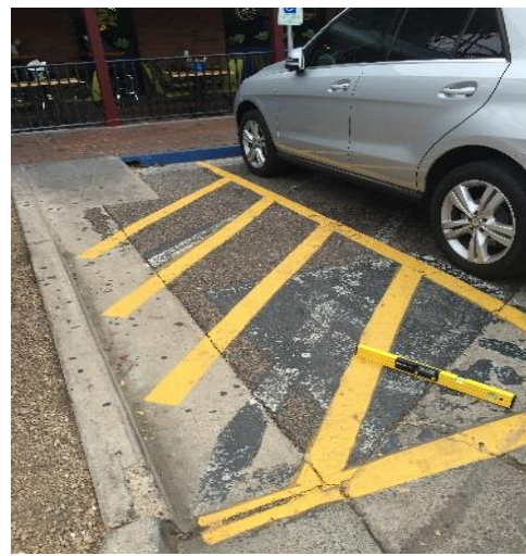
Figure 7: 4 th St. – Curb ramp within access aisle
