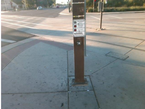
Figure 4: Pedestrian Push Button
