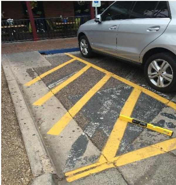
Figures 10 and 11: W. 4 th St. – 4.9% slope within parking spaces
