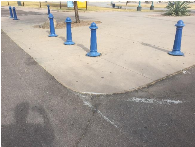
Figure 17: Change in level at access point
