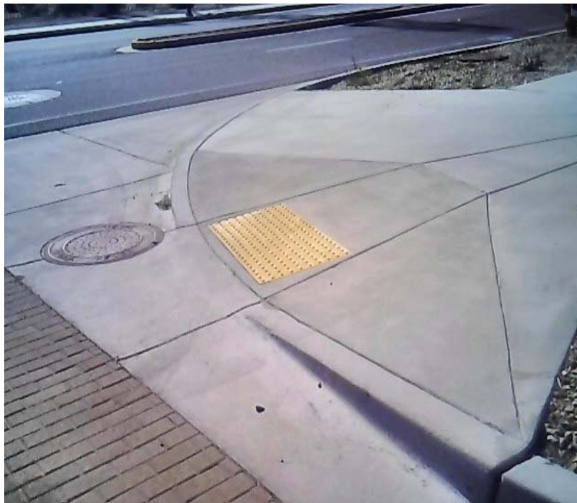
Compliant Perpendicular Ramp
