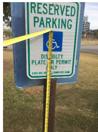
Figure 18: Parking signs are too low.
