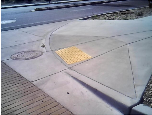
Figure 2: Compliant Perpendicular Ramp
