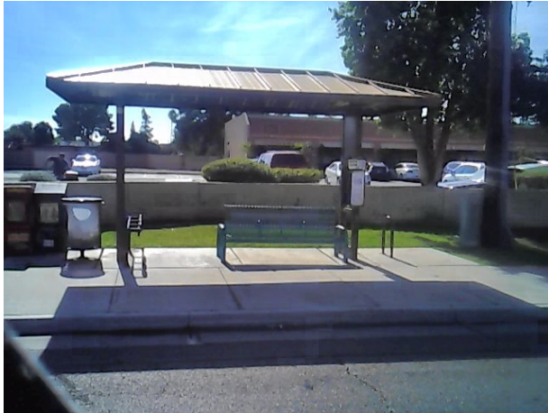
Figure 4: Compliant Transit Stop
