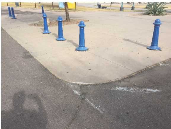
Figure 17: Change in level at access point
