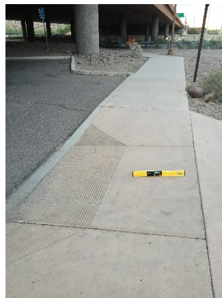
Figures 25 and 26: Curb ramp slope 10.9%
