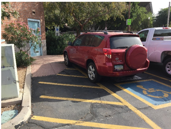
Figure 14: City Hall West – Curb ramp within access aisle
