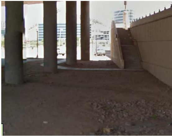
Figure 23: No accessible route from N. Mill Ave.
