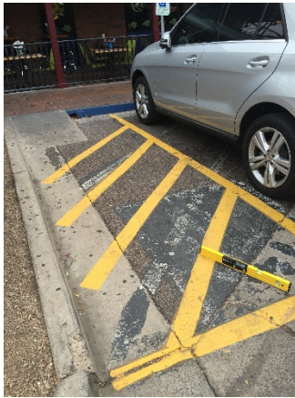
Figures 10 and 11: W. 4 th St. – 4.9% slope within parking spaces
