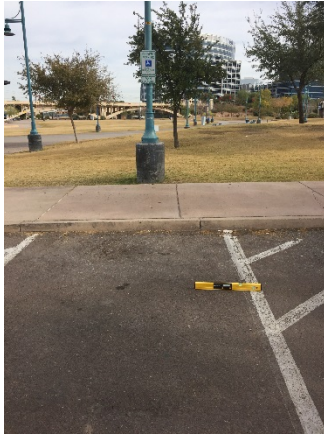
Figures 19 and 20: Slopes greater than 1:48 within accessible parking
