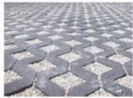
POROUS CONCRETE DECOMPOSED GRANITE FILL
