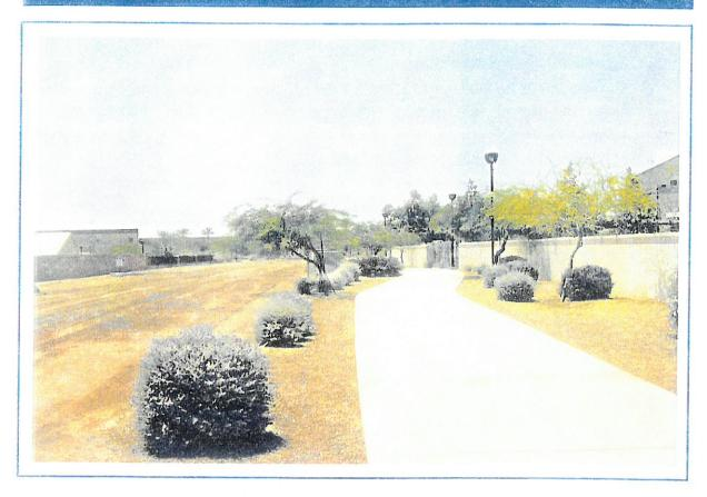
The City of Tempe endeavors to provide a safe, attractive, and functional multi-use path system for residents and visitors in the City. The recommended design standard for the paths is a 25-foot wide easement with a 12-foot wide concrete path and landscaping and lighting in the remaining 13 feet. Lighting shall comply with City of Tempe lighting standards. Additionally, the City strives to incorporate art elements into these projects.
