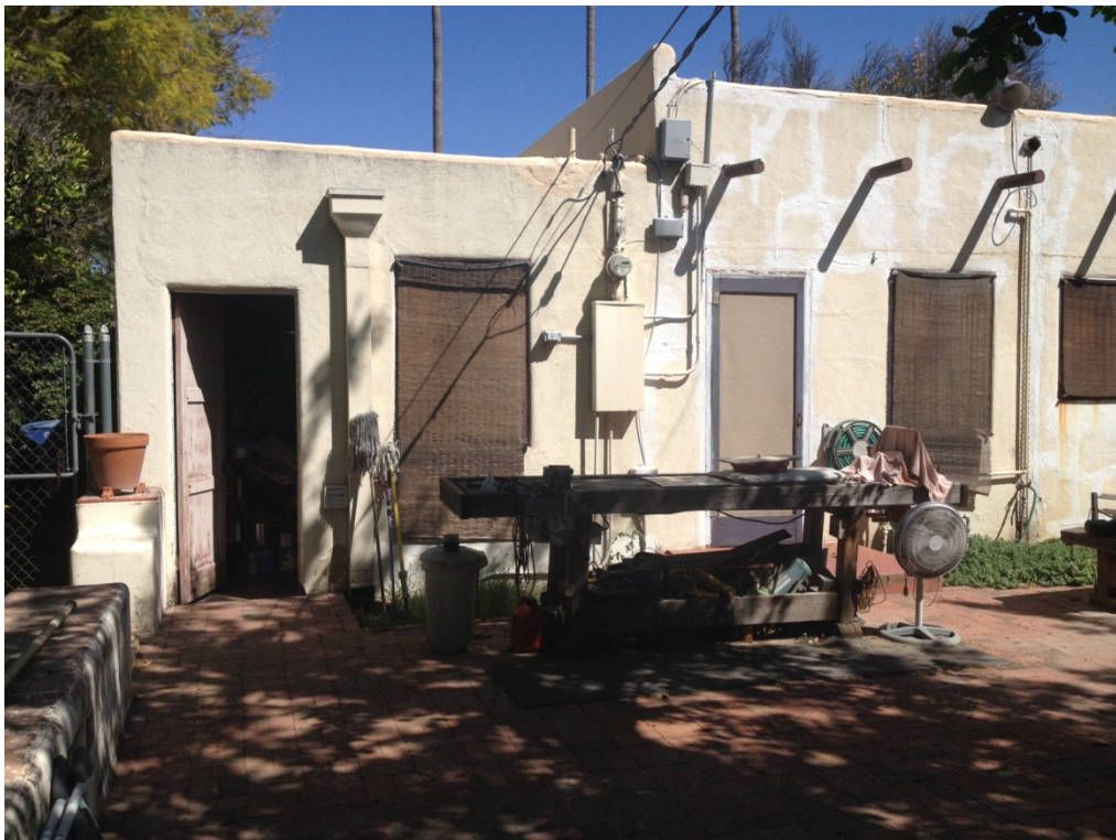
Lindstrom (Nucci) House – Northernmost portion of rear (west) elevation
