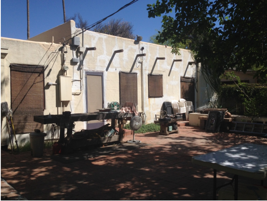
Lindstrom (Nucci) House – Rear (west) elevation
