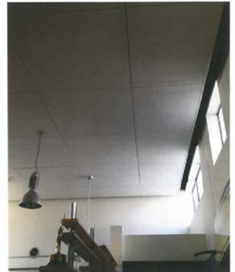
Interior Clerestory Windows
