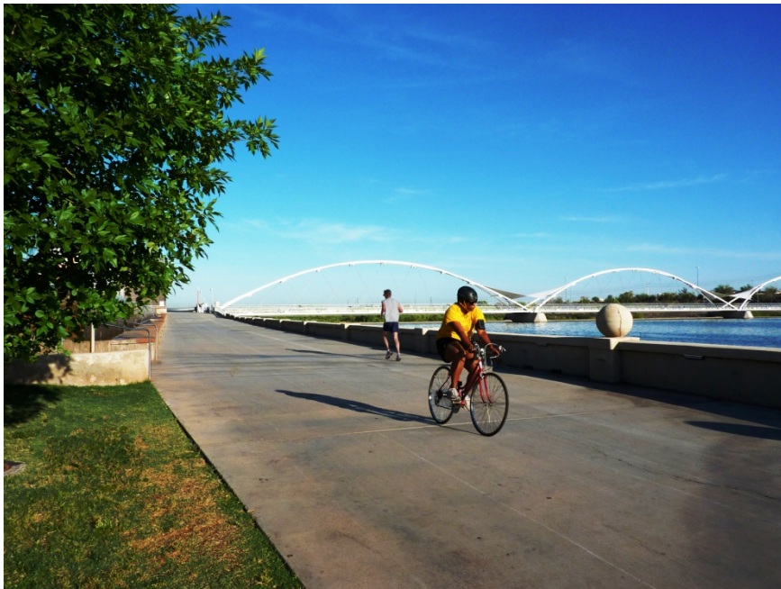
Downstream Dam Images
