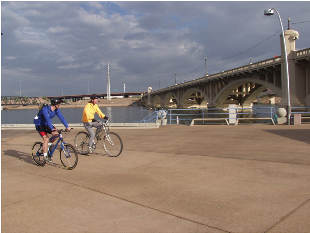
Undperass @ Mill Avenue
