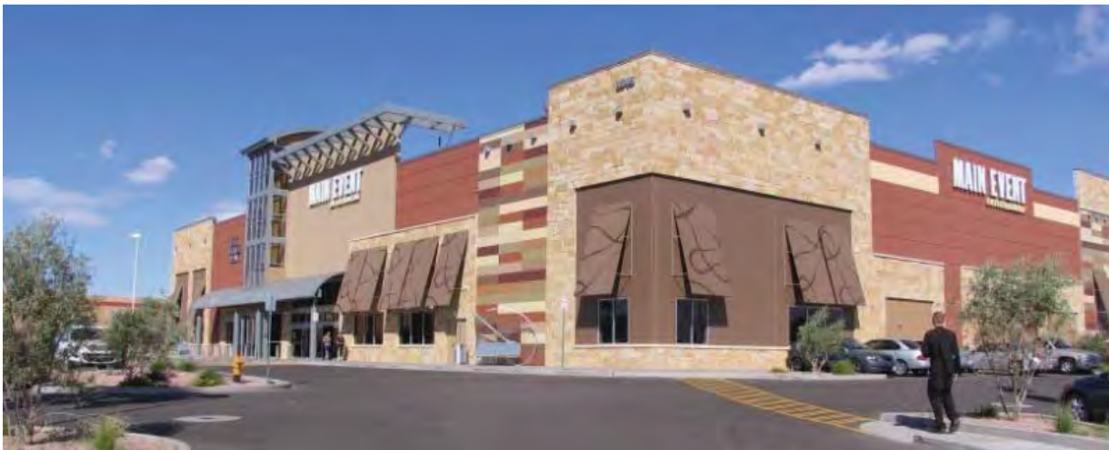
Main Event south west elevation looking north
