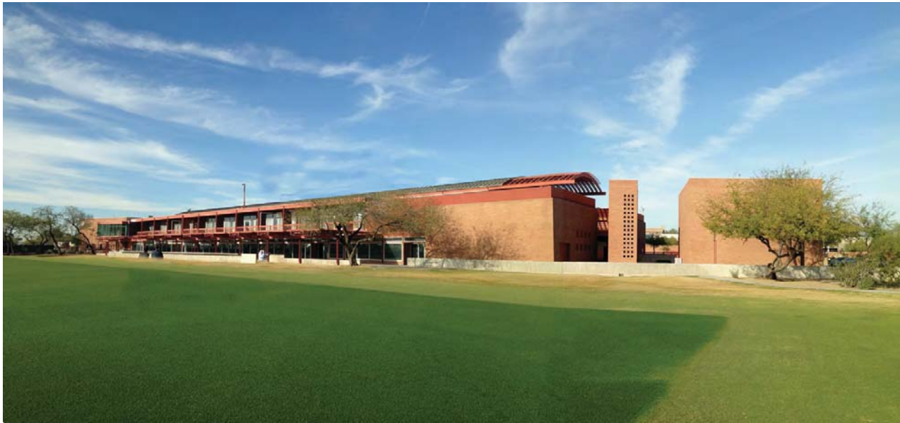
BEFORE BUILDING ADDITION
