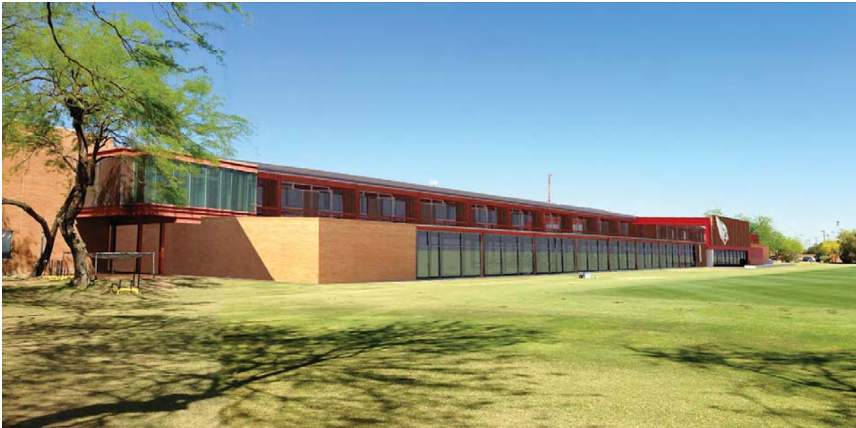
AFTER BUILDING ADDITION
