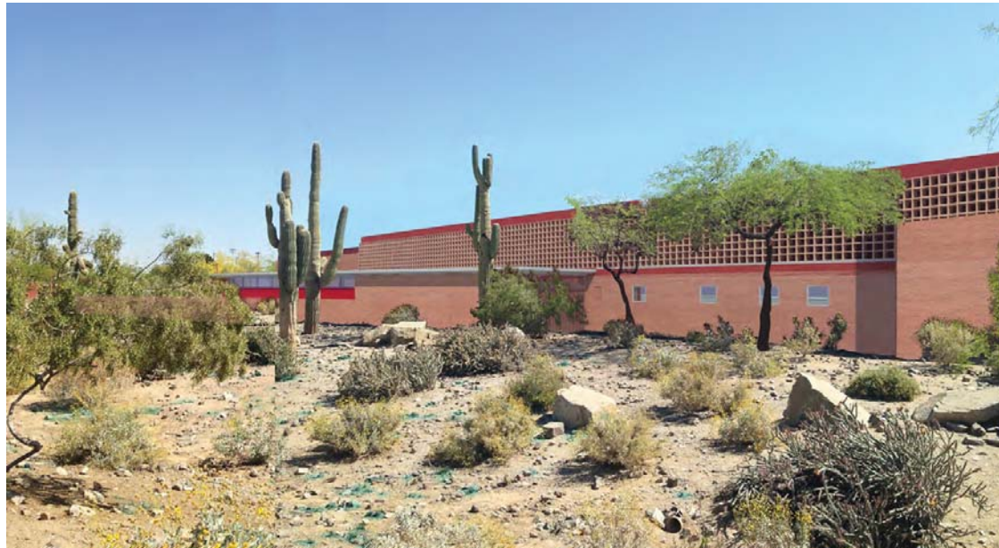
AFTER BUILDING ADDITION
