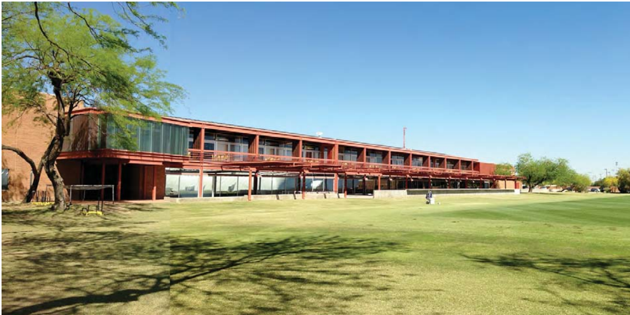
BEFORE BUILDING ADDITION
