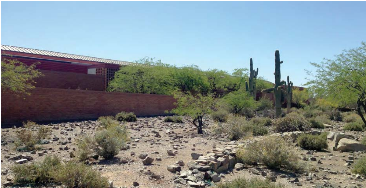
BEFORE BUILDING ADDITION
