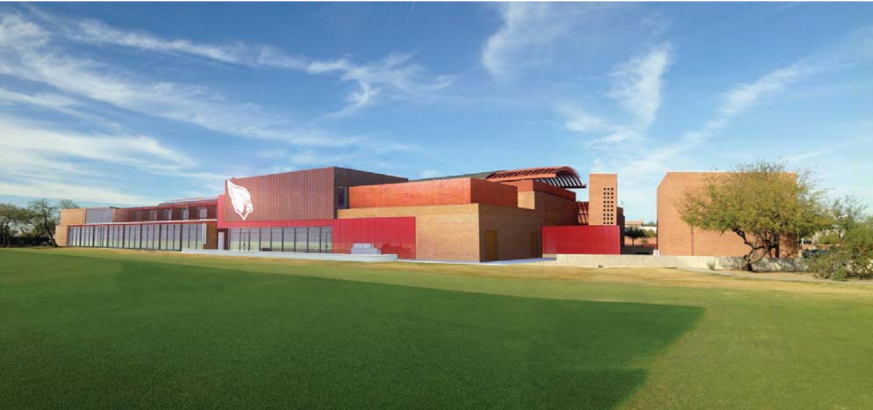
AFTER BUILDING ADDITION
