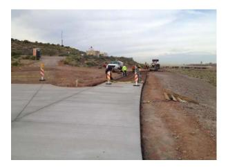
The purpose of this project is to construct a 10-foot wide concrete multi-use path with lighting and safety railings adjacent to Rio Salado (Salt River) between Priest Drive and the City of Tempe boundary with Phoenix just east of SR 143/Hohokam Freeway.
