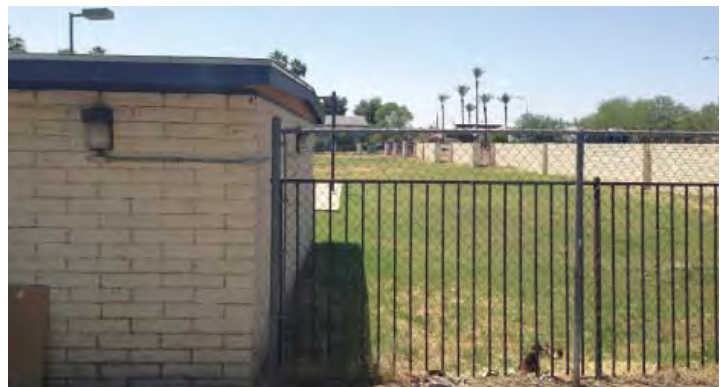
4 WEST - ALLEY FRONTAGE
