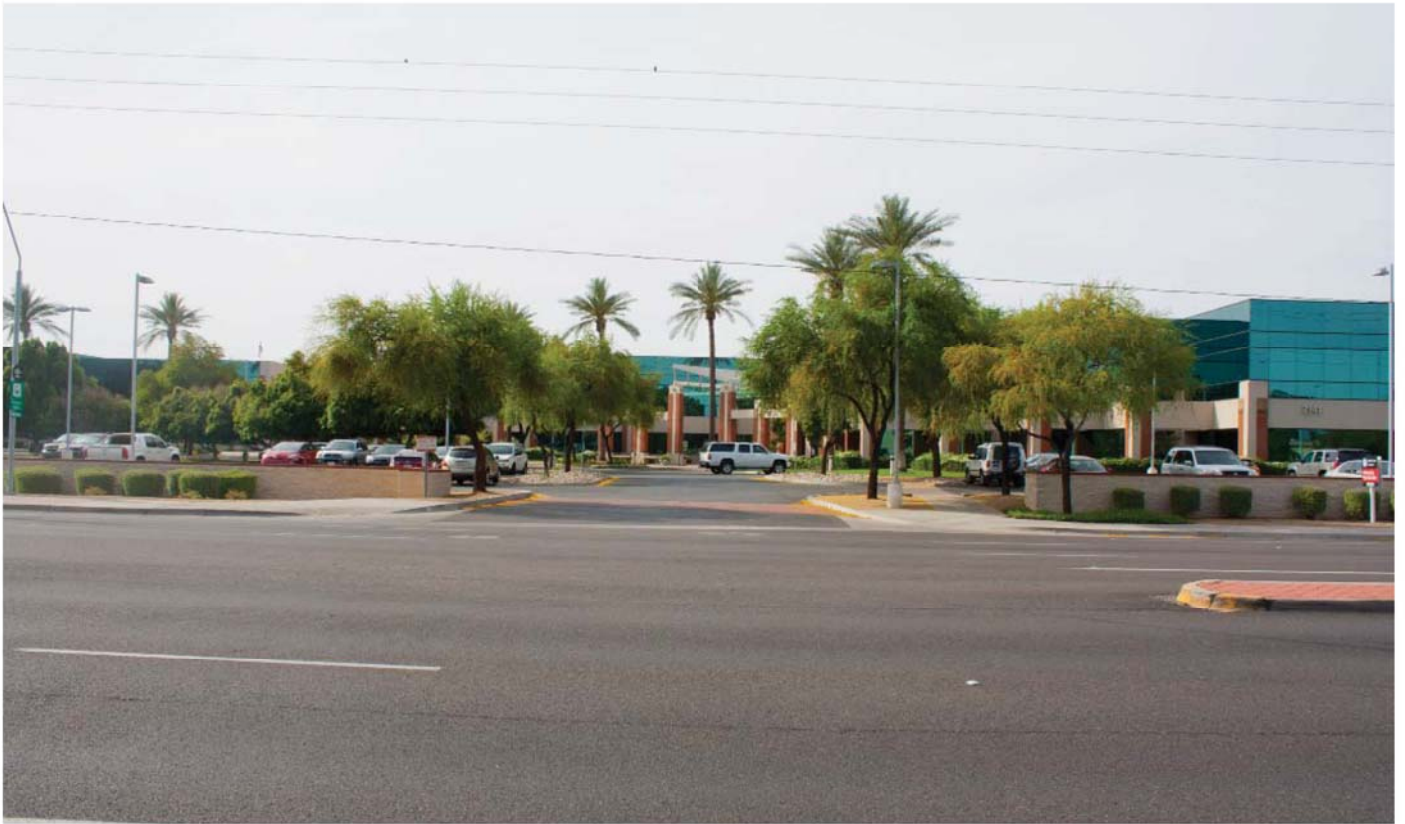
19 SOUTHWEST COLLEGE OF NATUROPATHIC MEDICINE, BROADWAY ACADEMIC BUILDING 2156 E BROADWAY RD, TEMPE, AZ FACING SOUTH, FROM S. EDGE OF SITE DATE: APRIL, 2013
