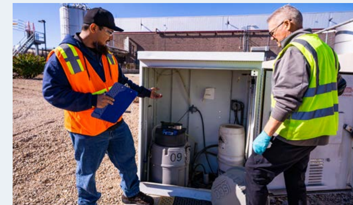
Environmental Compliance Inspectors conduct industrial inspections to ensure cross connection control, stormwater and wastewater code requirements are met.
