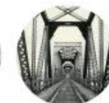
LITHO #9 Railroad Bridge
