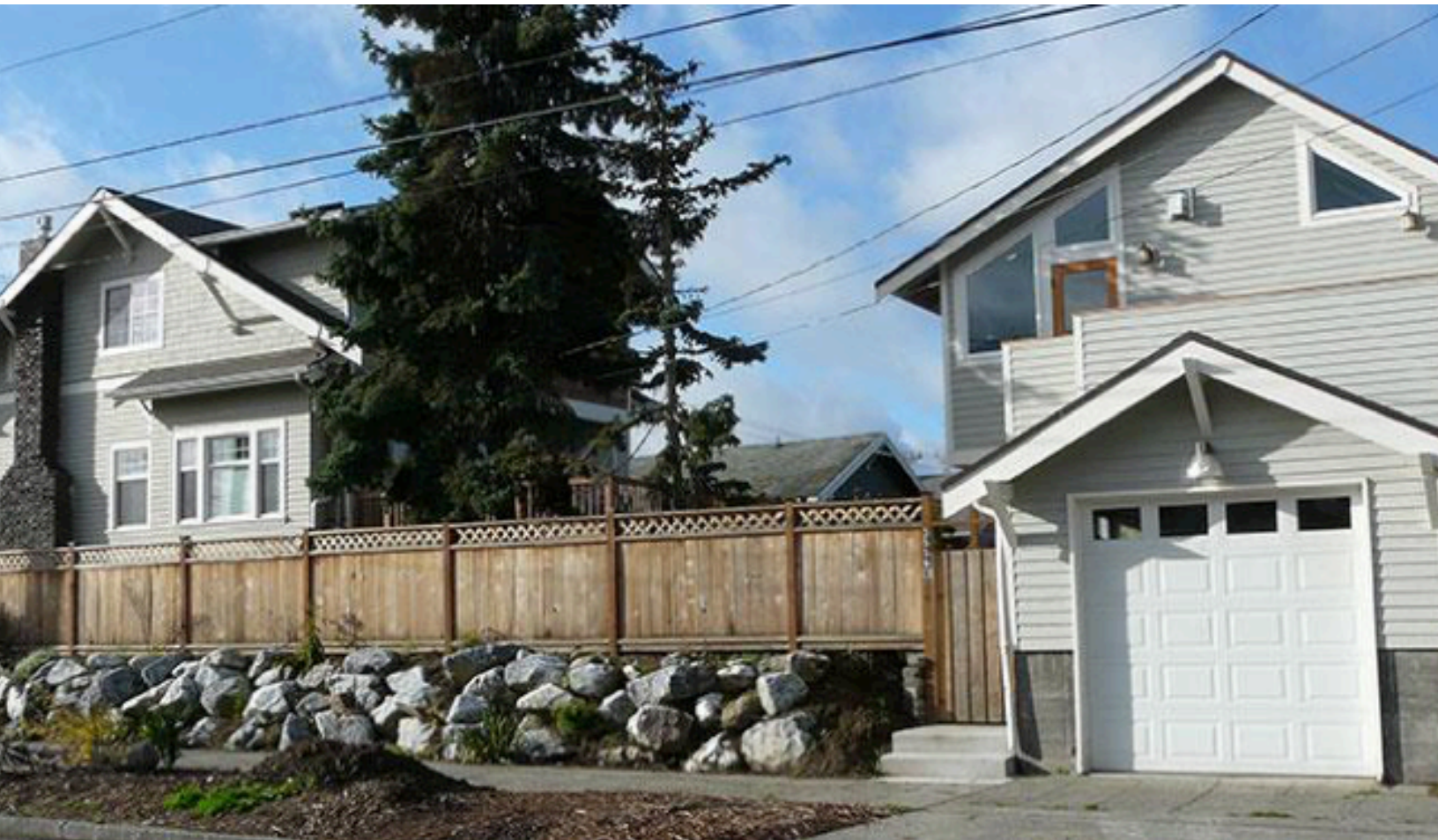
Seattle ADU, photo credit: City of Seattle.
